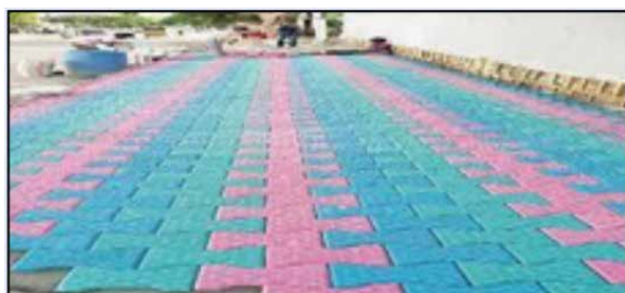
Figure 9.12 Pavement constructed using recycled plastic tiles (MoHUA, 2019)
